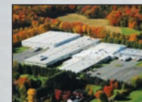
South Deerfield, MA office and manufacturing plant
