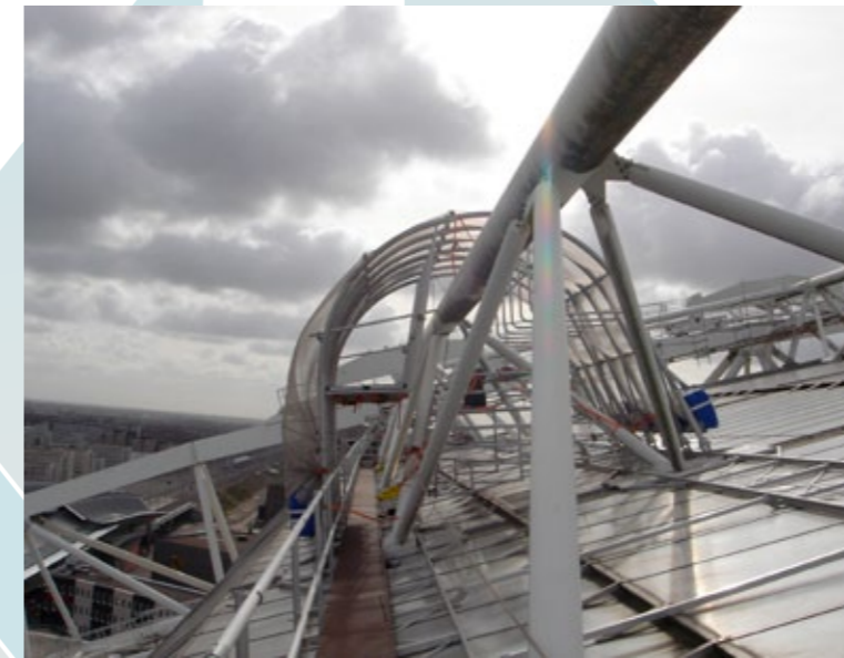
special Construction for maintenance to the roof of Ajax Arena Stadium
