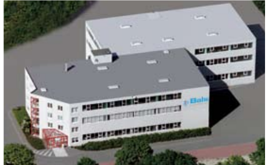
New plant in Freiwalde (Brandenburg)
