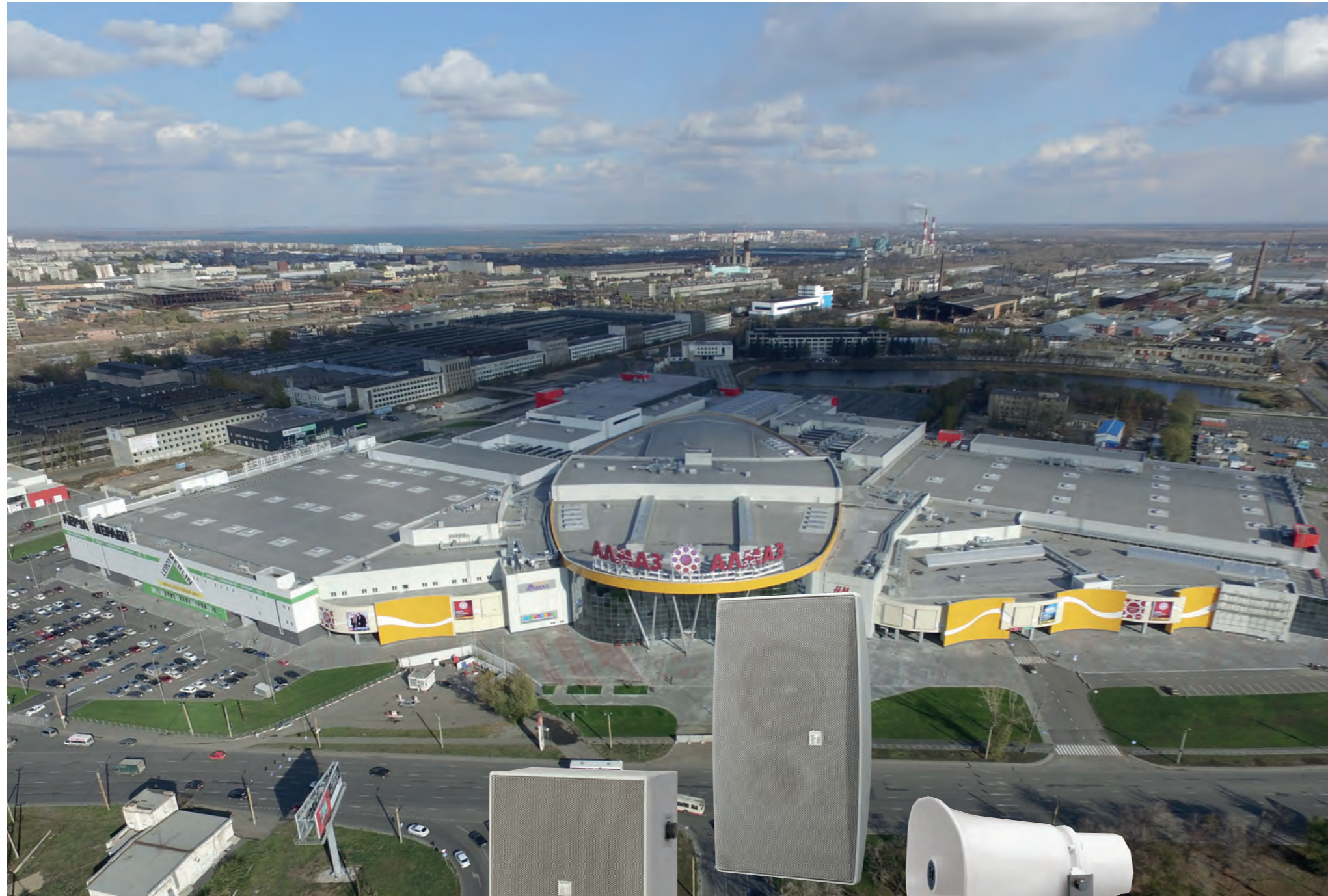
More than 3,200 TOA speakers were installed in the Mega Mall in Chelyabinsk, a Russian city in the Ural region.
