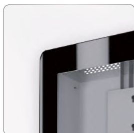
High level finishing
